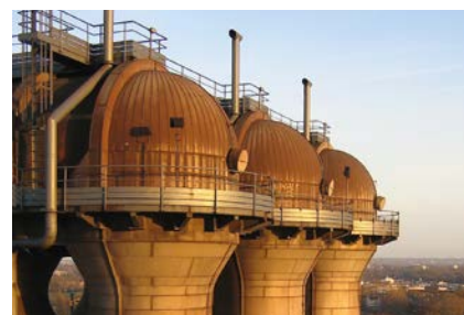
Blast furnace / stove dome
