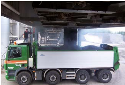
Asphalt and concrete mixing
